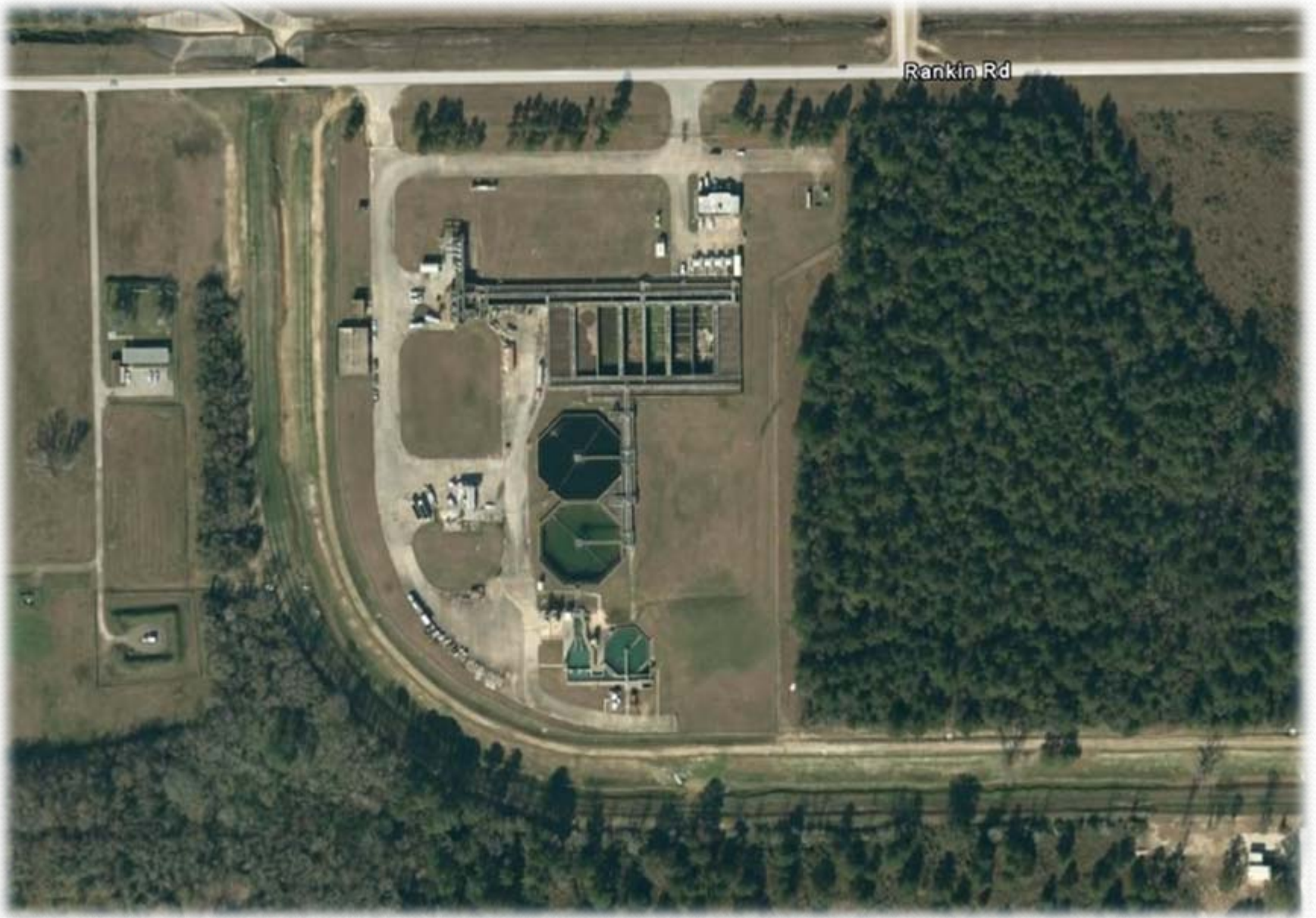
IAH Wastewater Treatment Plant – Houston, Texas
