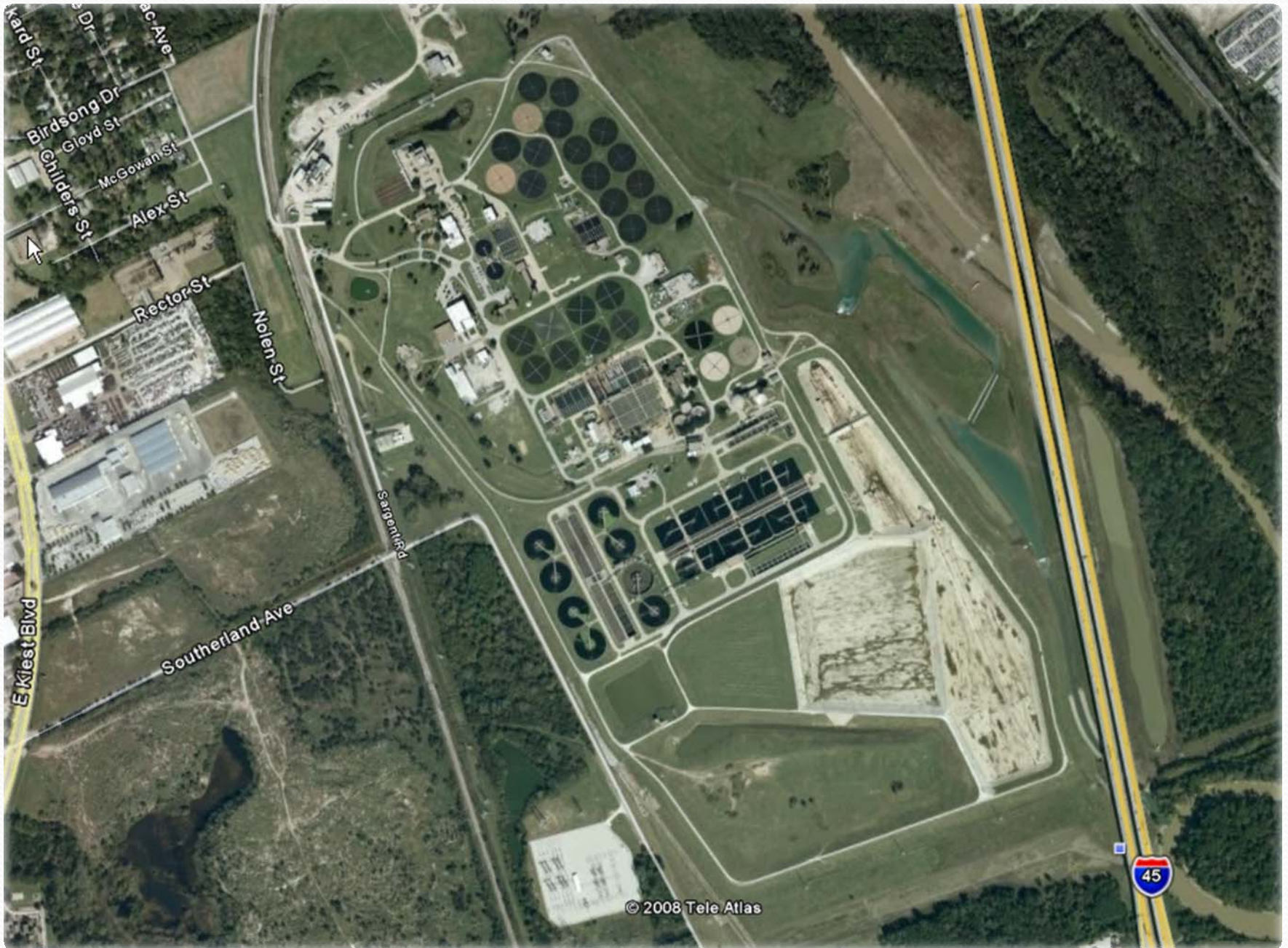
Dallas Central Wastewater Treatment Plant – Dallas, Texas
