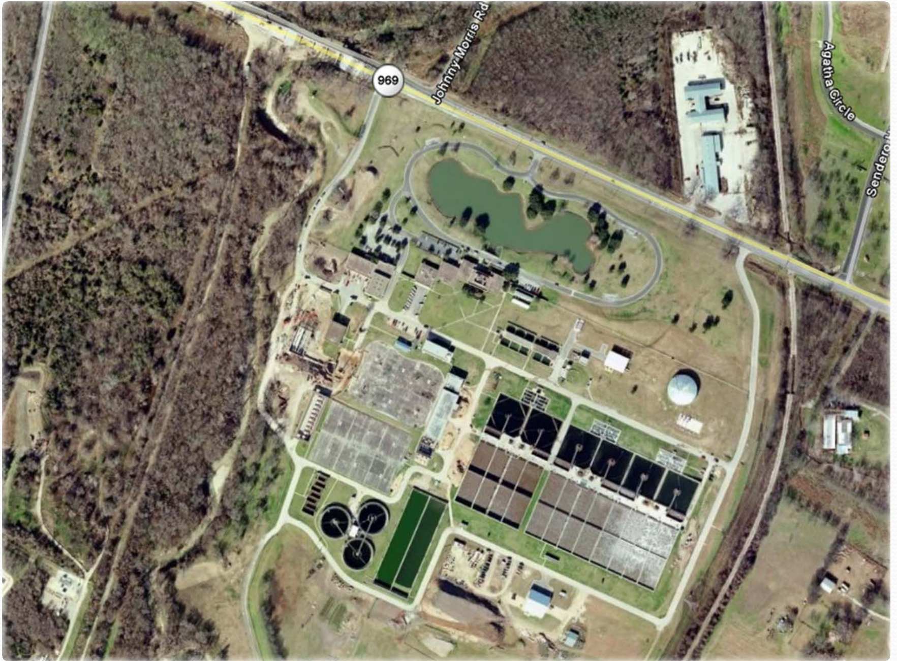
Walnut Creek Wastewater Treatment Plant – Austin, Texas
