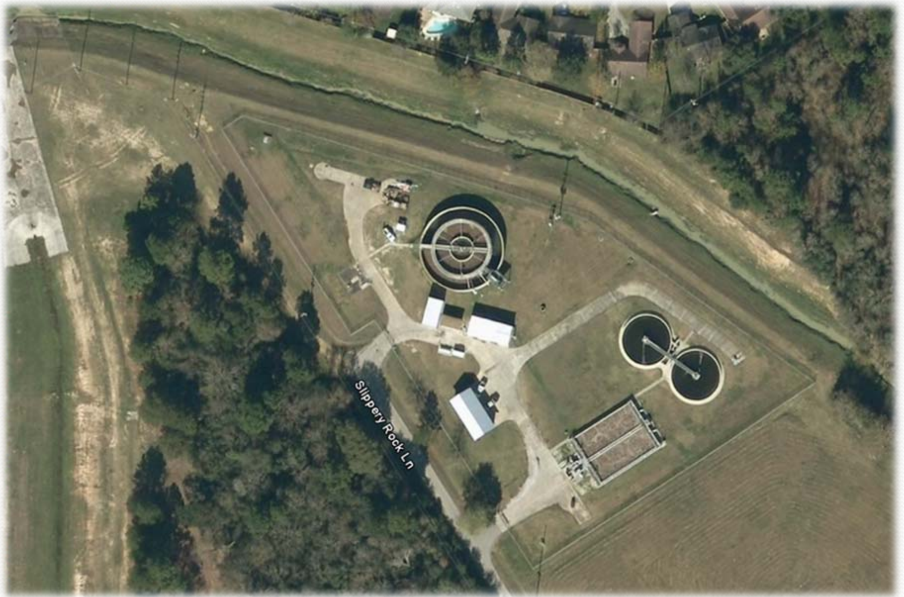
Bridgestone MUD Wastewater Treatment Plant – Spring, Texas
