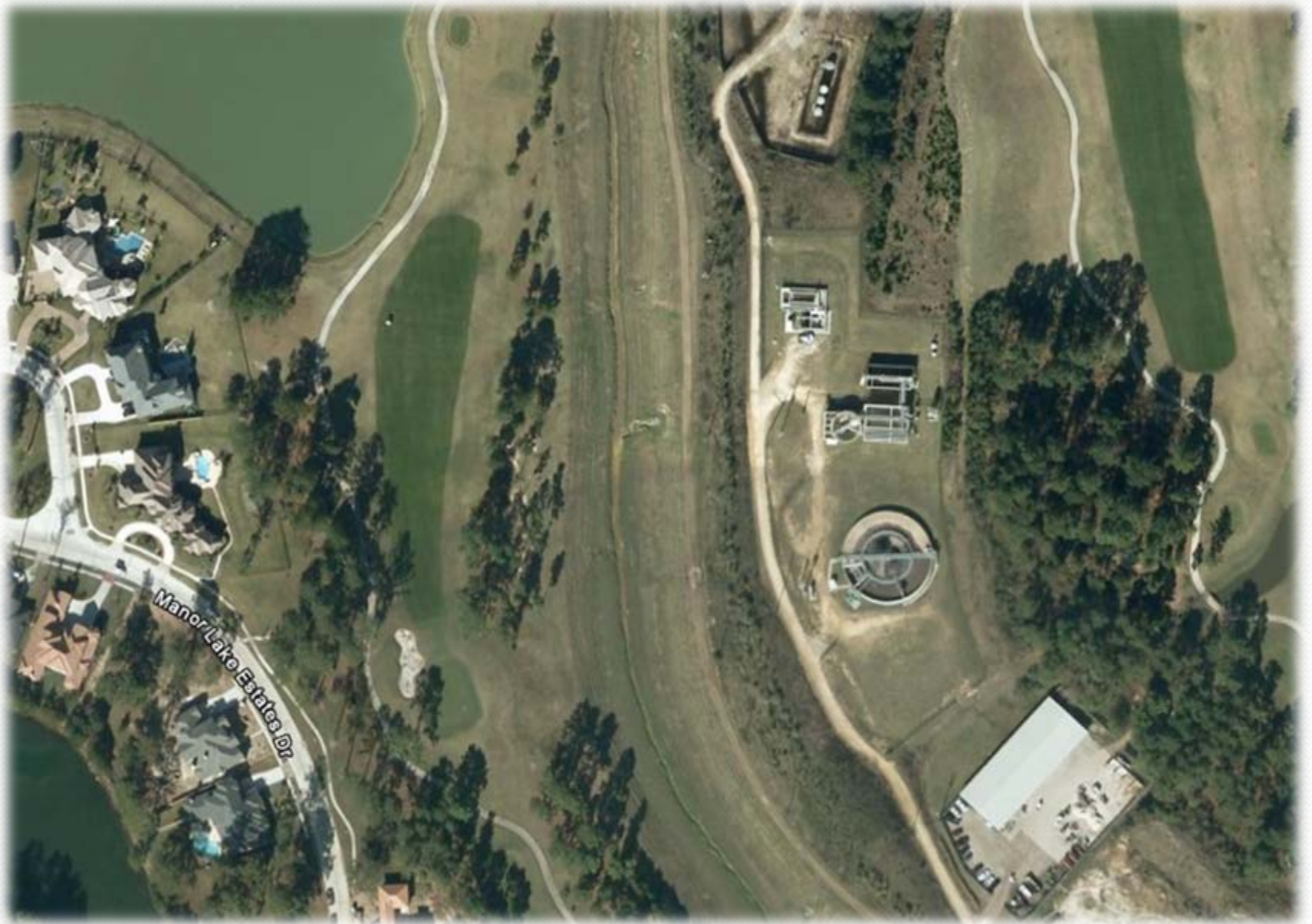
Harris County MUD 367/383 Wastewater Treatment Plant – Spring, Texas
